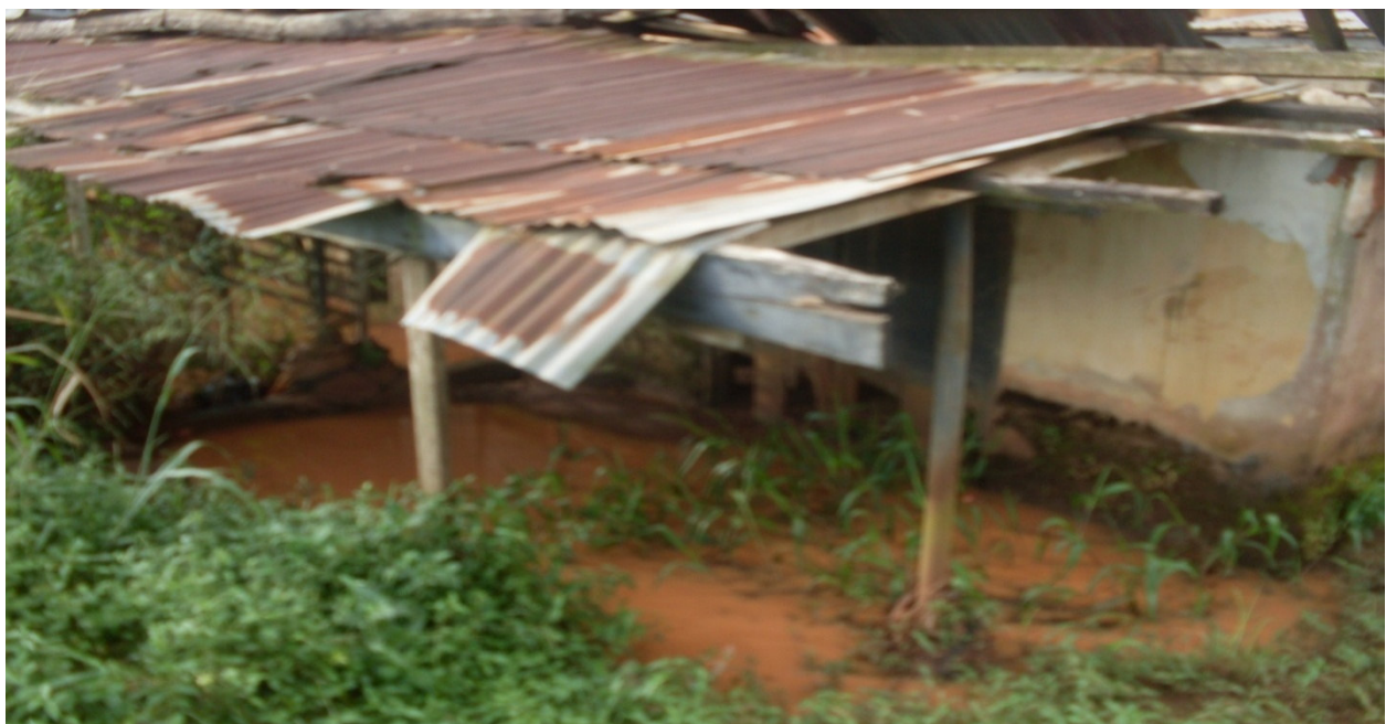
Figure 10. Abandoned residential house in flood area.
