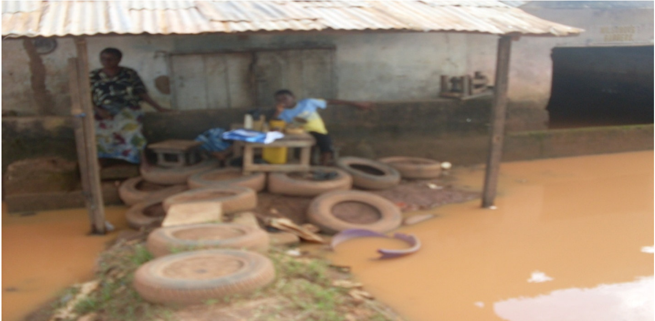
Figure 13. Raised walkway with old vehicle tires as a strategy for reducing erodibility.
